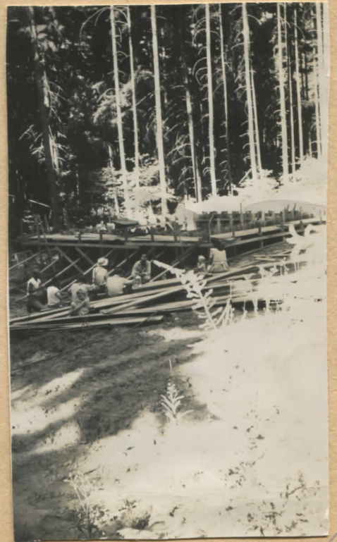
Building house on Romona
